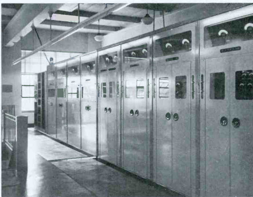
There are two 50-kw transmitters at WLW. In the foreground is the transmitter designed by Ronald J. Rockwell and built by station personnel. This is WLW's main transmitter and features an audio response from 20 Hz to 20 kHz. Just beyond this transmitter is a completely rebuilt Western Electric unit.
