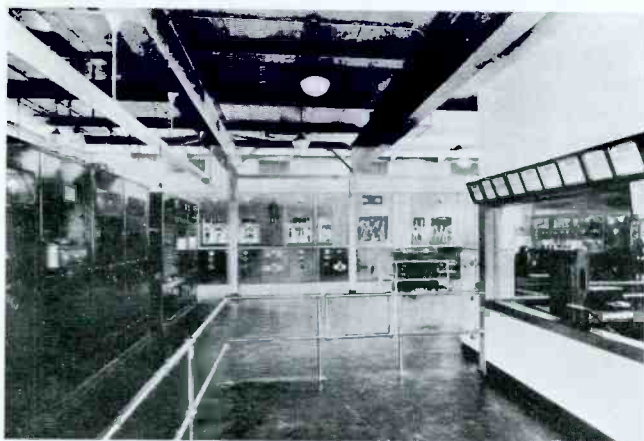
This view shows the WLW transmitter building as seen from the front entrance. The 50-kw exciter appears at the left, the 500-kw amplifier-modulator is in the background, and the audio control room is at the right. Circa 1934.
